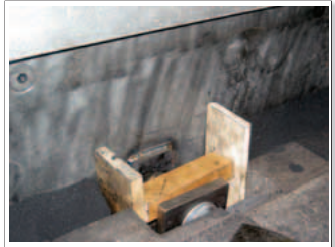
Figure 5. Hanging system with the formwork to pour in the Sigrí RST16.
